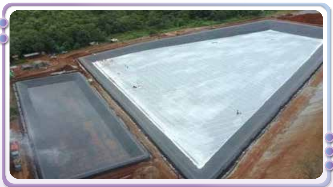
Constructing additional safe landfill with water storage and observation ponds
