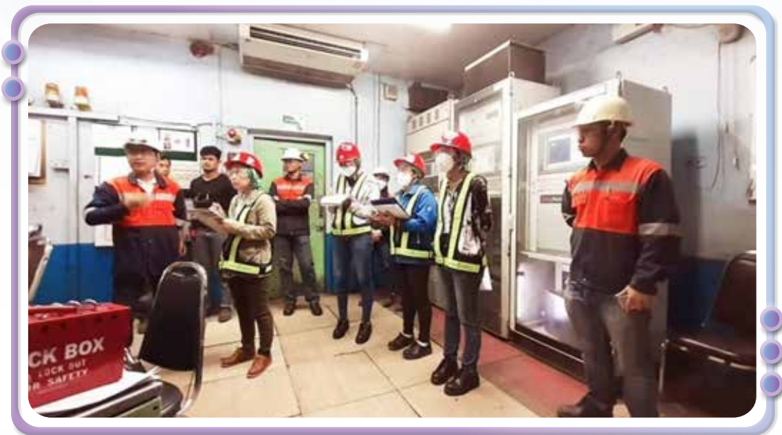
Verification in the joint operating area of the CSR-DPIM Network Project
